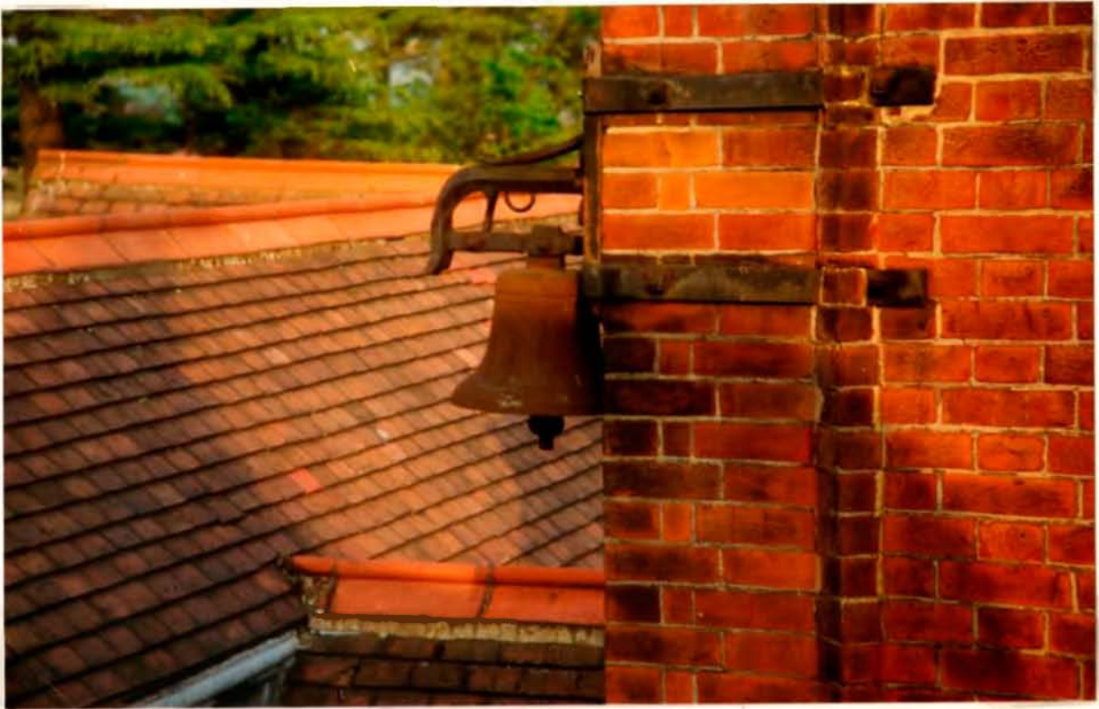
The roof-top Fire Bell.
