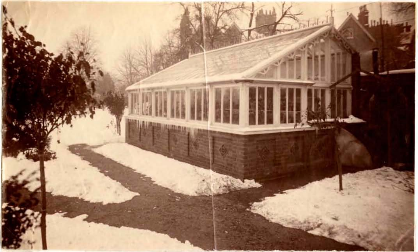
The elegant Greenhouse. Patterns built into the brick base. Ornamental eaves and roof-ridge.
