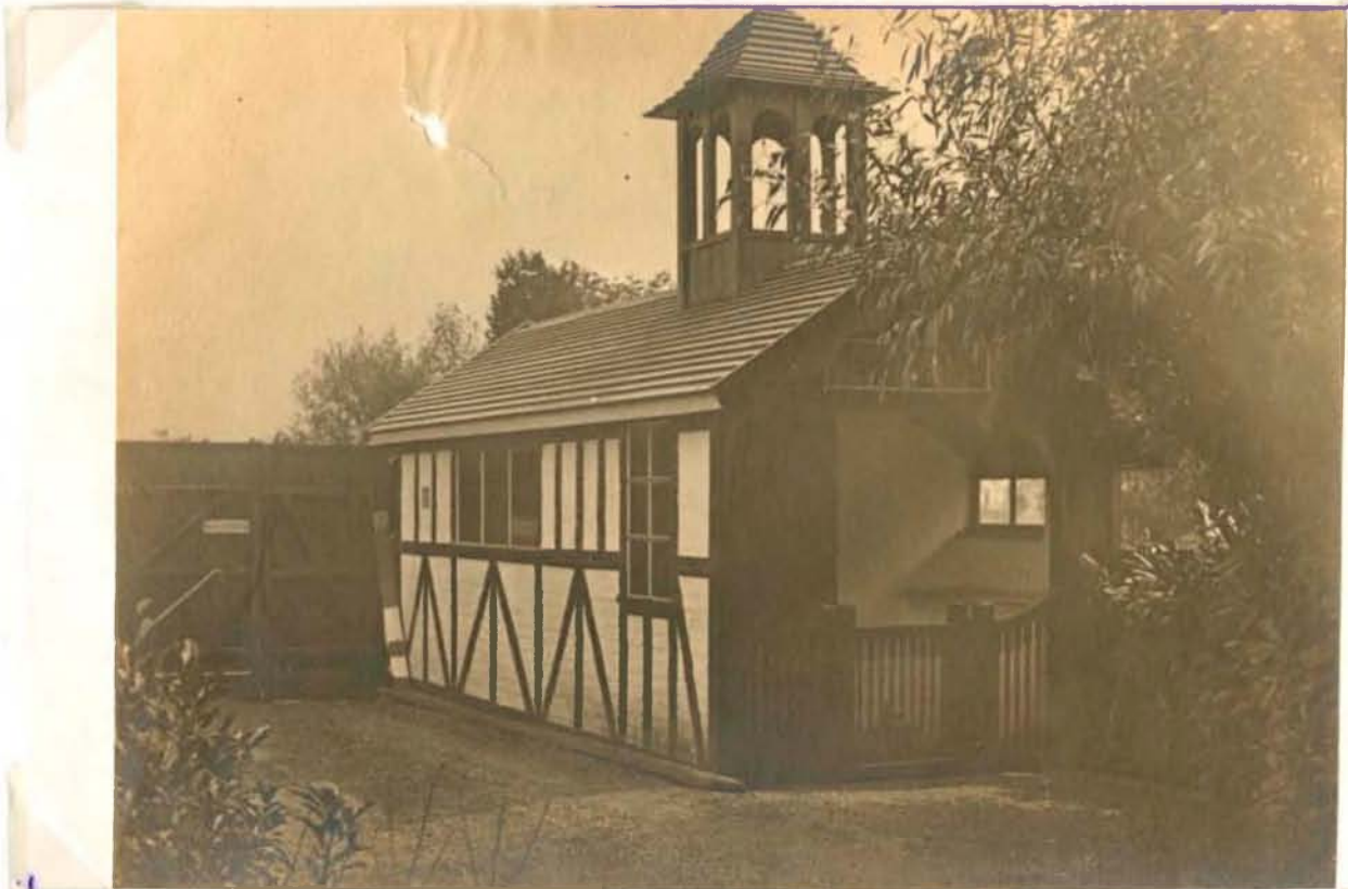
Front-part, The Potting Shed. Rear-part, The original Dairy. Situated by the lower gate at the South-East corner of the Estate on Datchet Road. (The gate closest to The Myrke).
